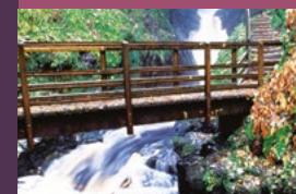
Glenariff Road, BT44 0QX near Waterfoot
